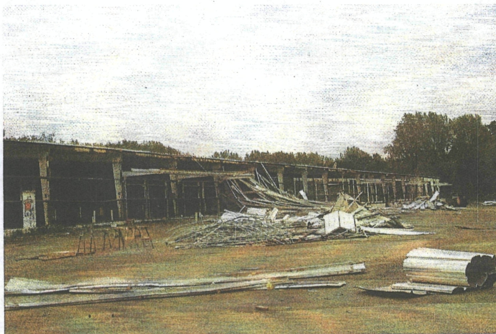
Dico Building 4/5 demolition; view to the south 9/19/07
