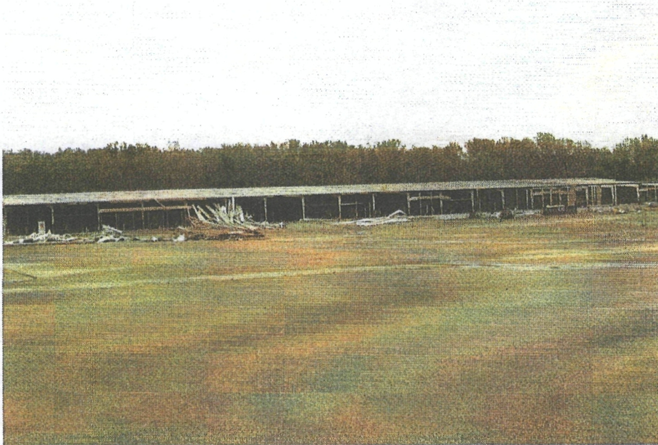
Dico Building 4/5 demolition; view to the east 9/19/07
