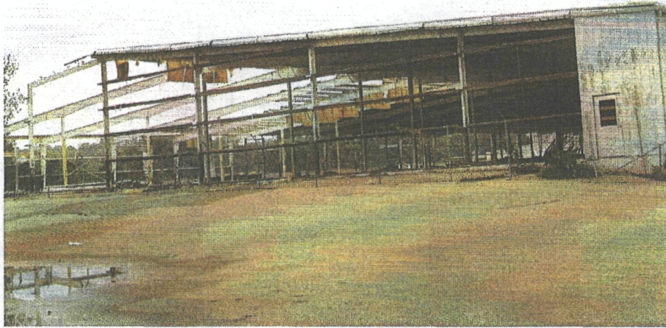
Dico Building 4/5 demolition; view to the northwest 9/19/07
