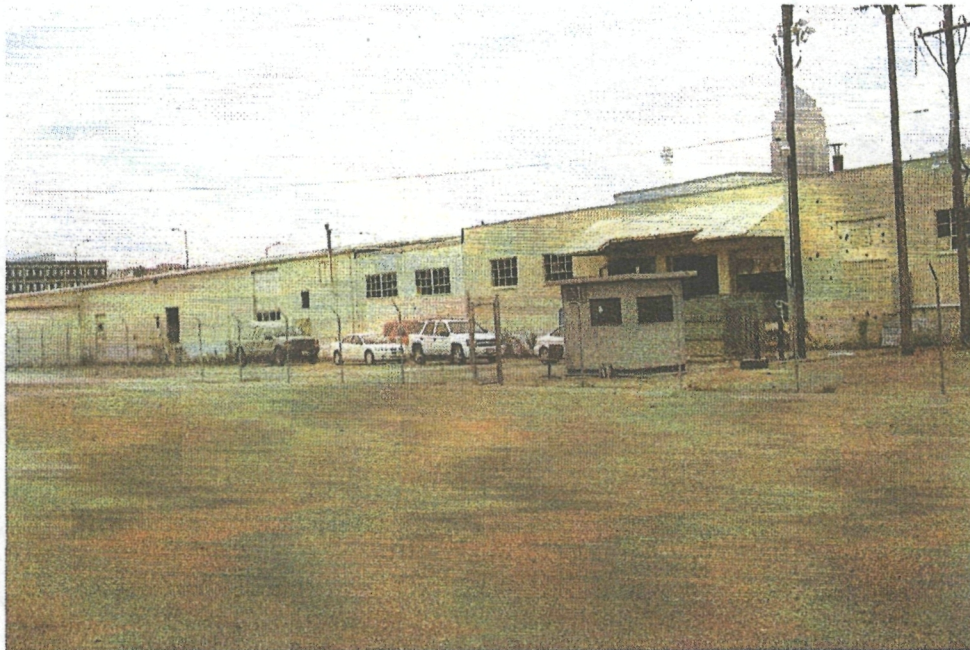
Dico Production Building; view to the east Shows new security fencing and guard shack 9/19/07
